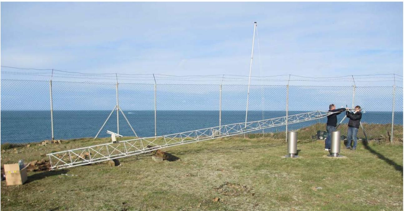
*Guernsey Met Office staff lower a 10 metre wind mast at Chouet in order to service and maintain the instrumentation. The wind data from this installation is used for research into the island’s potential for generating electricity from wind power and is passed on to the Department of Commerce and Employment. Photo credit: Martin Crozier*
